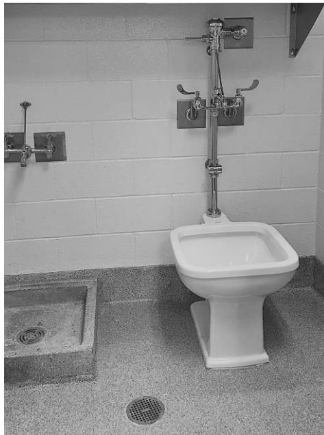
Example of a janitorial closet with a clinical sink for disposal of feces.
